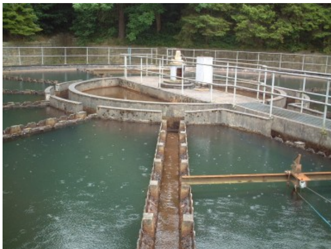
Figure 2: Solids contact unit for water clarification
